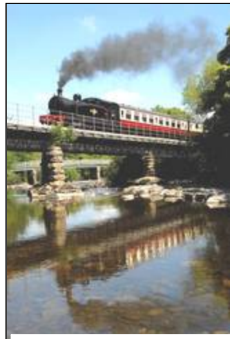
Broadwood Bridge June 2011
